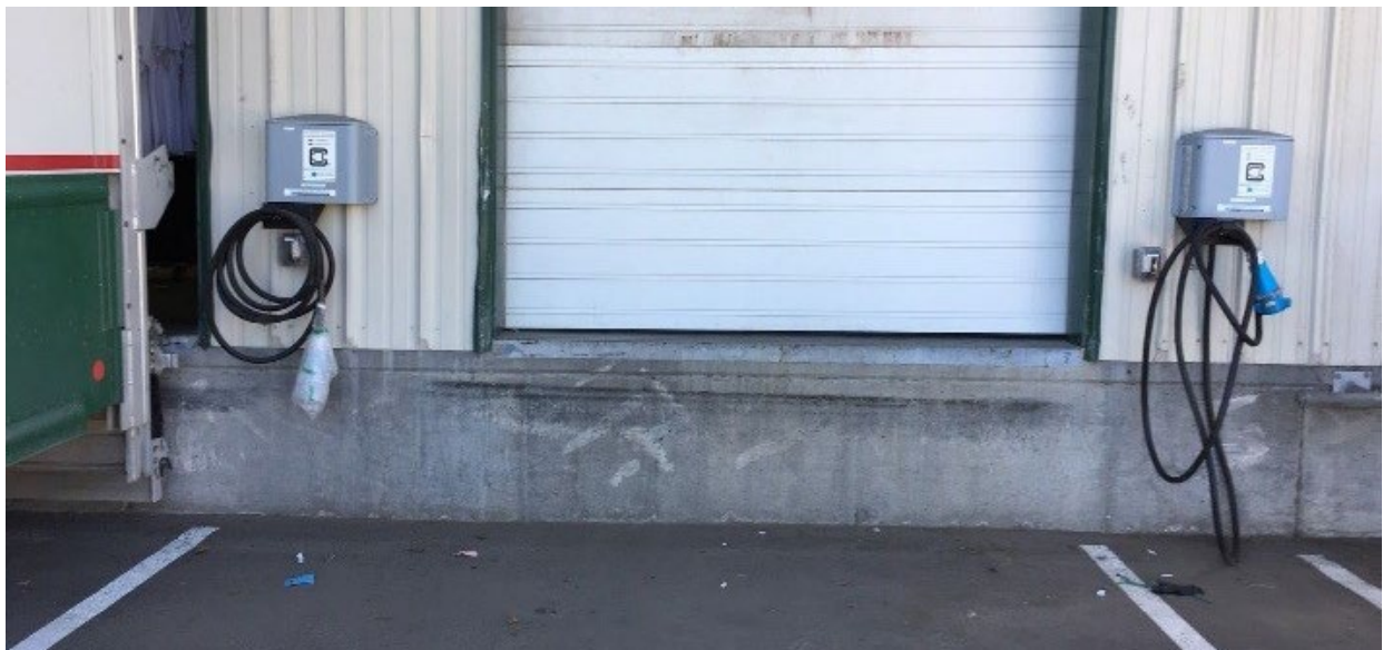
Stockton EVSE Installation
