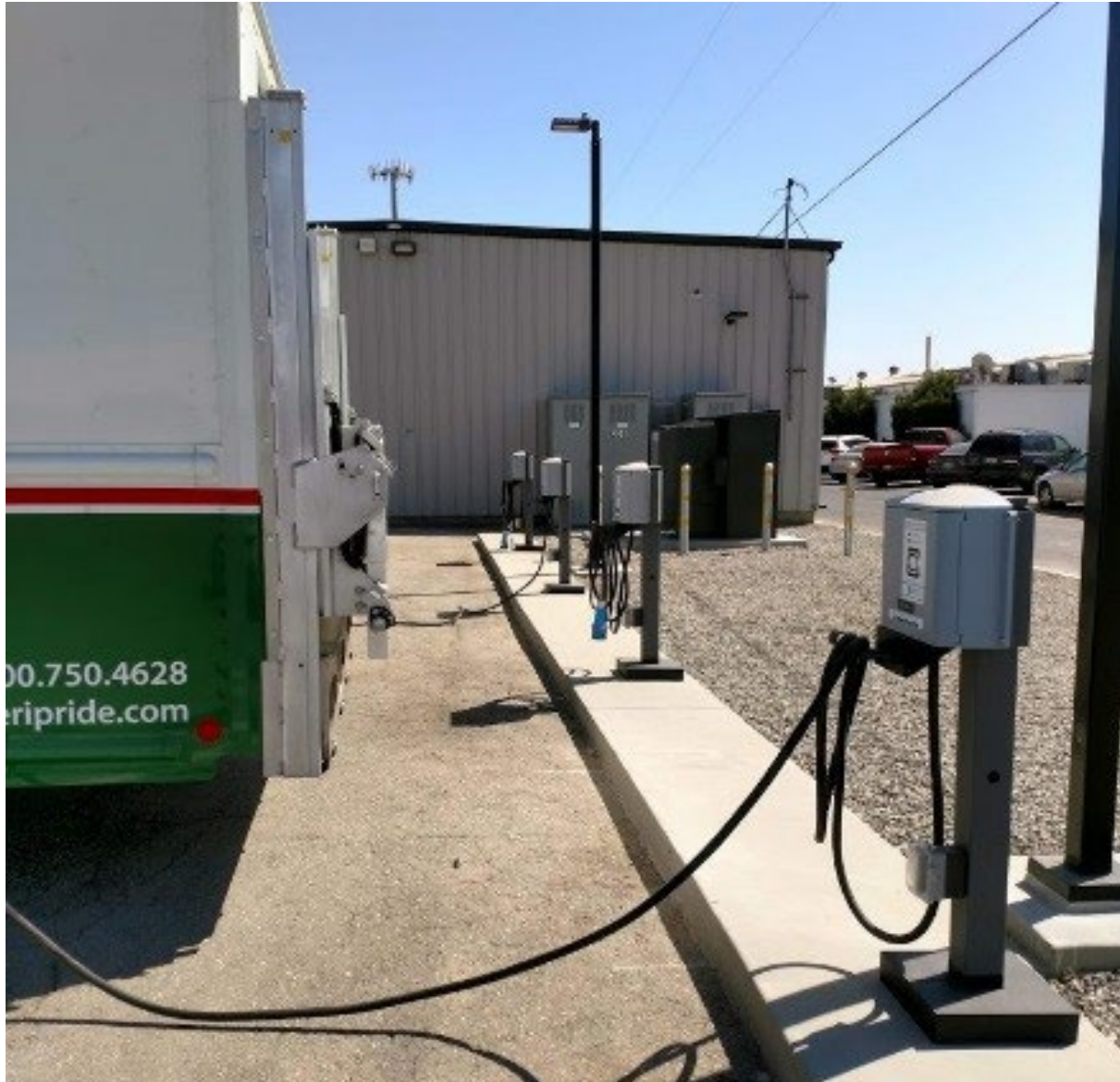
Bakersfield EVSE Installation
