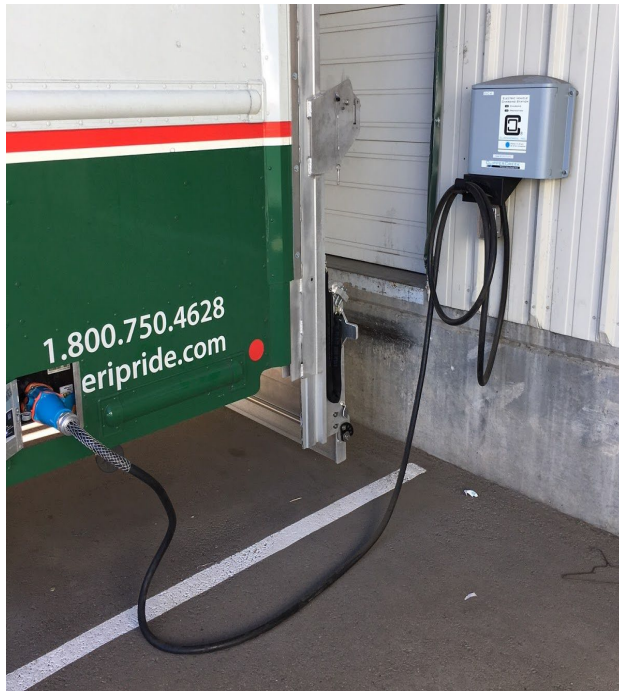
Stockton EVSE Installation
