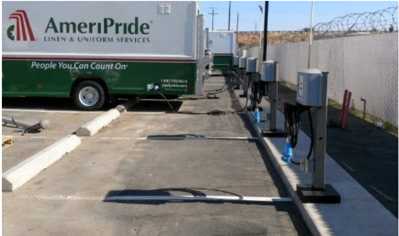
Fresno EVSE Installation
