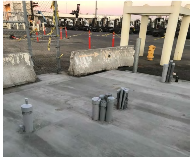
Figure 6: Concrete Cabinet Completed Work for Equipment
