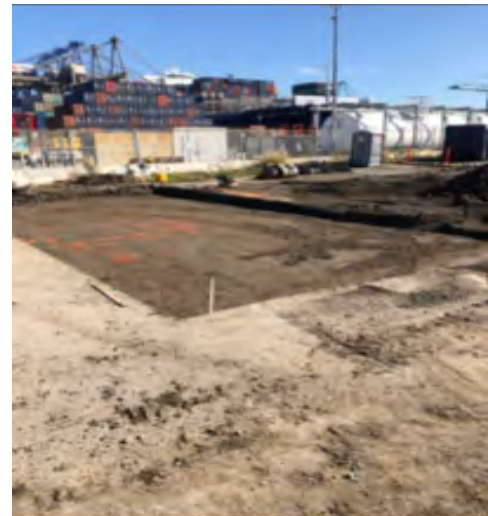
Figure 4: Excavation for Wireless-Charging Pad
