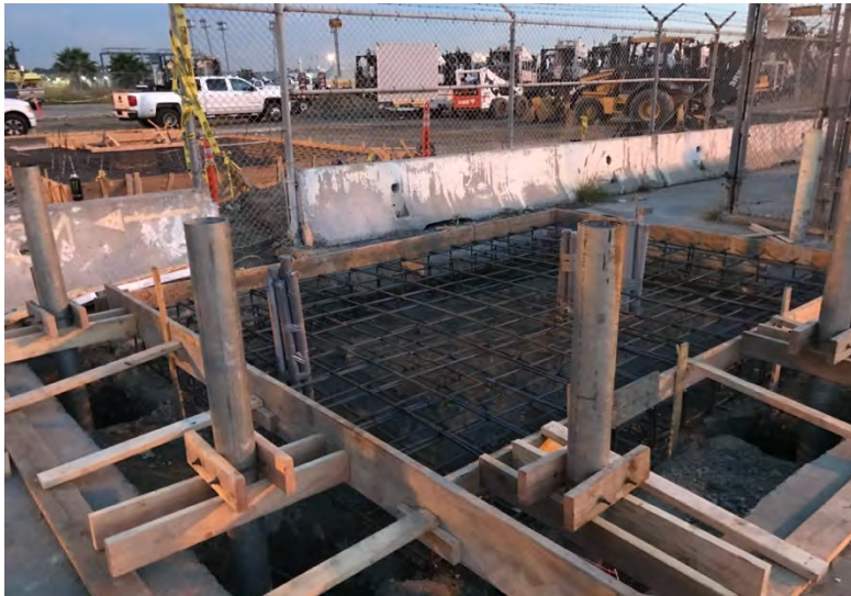
Figure 5: Concrete Equipment Rebar Set for Cabinet Pad
