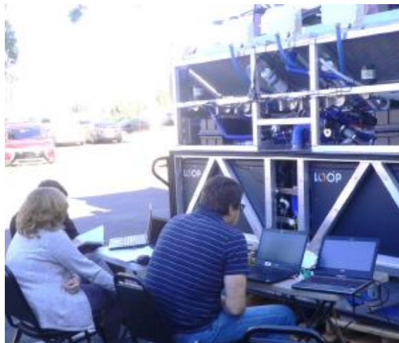
Figure 10 - The Loop fuel cell team commissioning the system for truck FC6
