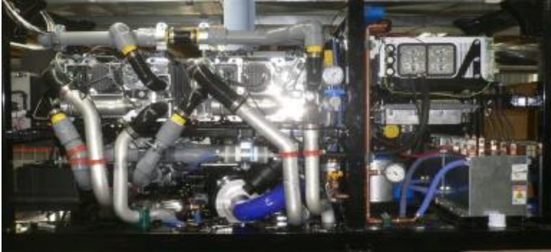
Figure 3 - Hydrogenics Fuel Cell System for Phase 1 FCFT Trucks
