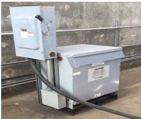
A TransPower EVSE with step down transformer and charging hardware box mounted to it. Credit: TransPower LLC
